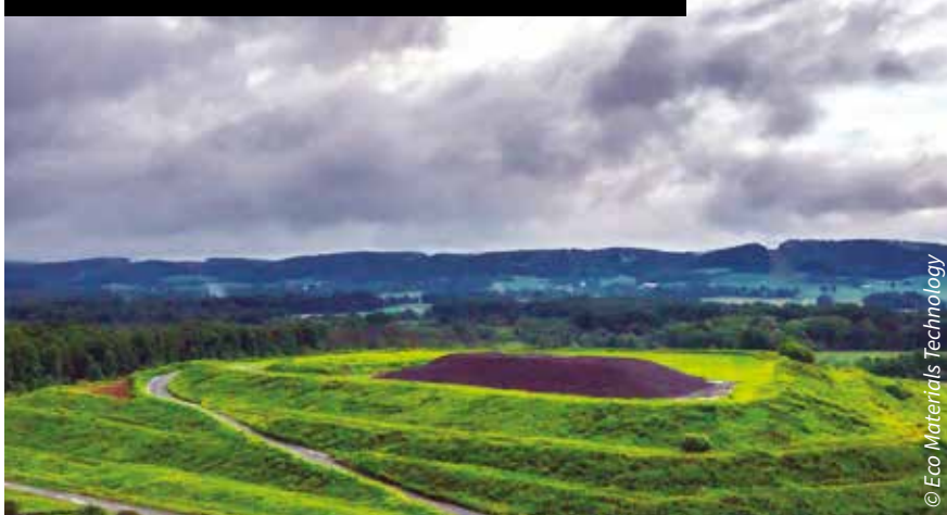
Eco Material's plant in Danville, Pennsylvania, which has provided fly ash used in concrete to repave roads around the state
