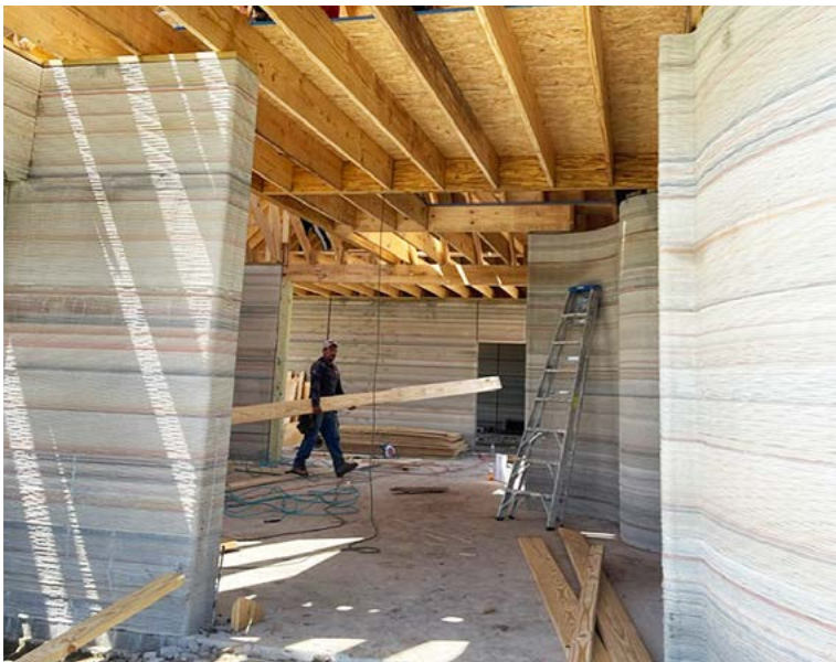
PozzoCem Vite 3D printing of a home
